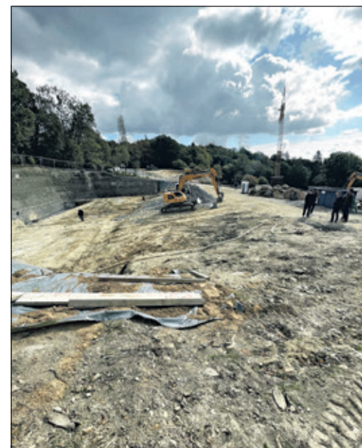
Where Indian rhinoceroses and Malayan tapirs will soon be making their rounds: The 18,000-square-meter construction site – crane included – already hints at the scale of the project taking shape here at a cost of 21 million euros. Foto: Glückert
