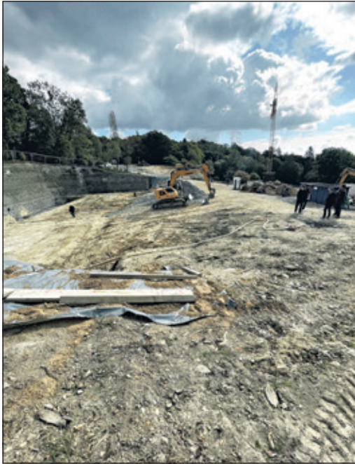
Where Indian rhinoceroses and Malayan tapirs will soon be making their rounds: The 18,000-square-meter construction site – crane included – already hints at the scale of the project taking shape here at a cost of 21 million euros. Foto: Glückert
